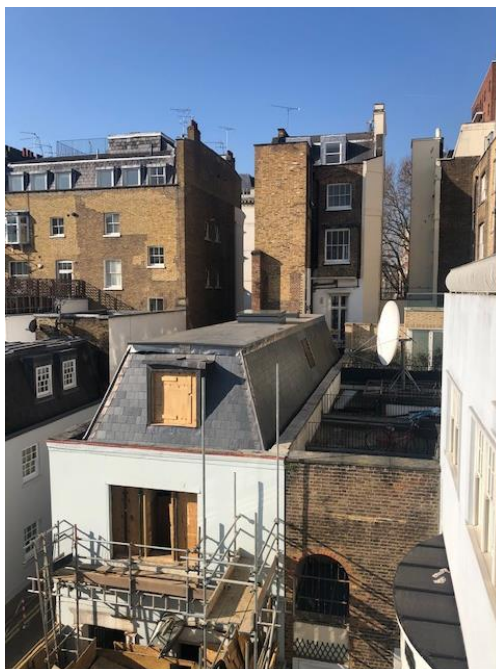
East elevation of mansard roof taken 27 February 2019
