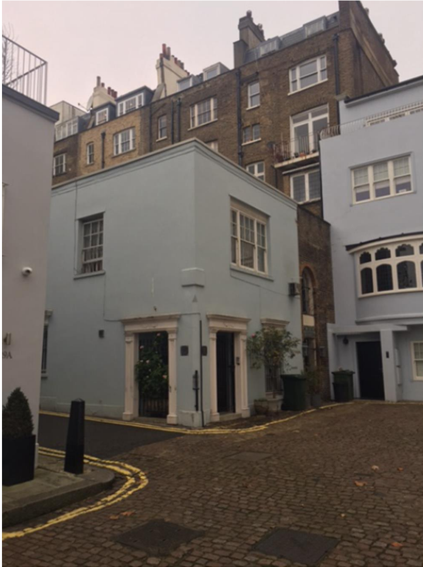
Application Site Before Works Commenced
