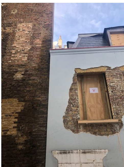
Dormer on west elevation taken 14 March 2019
